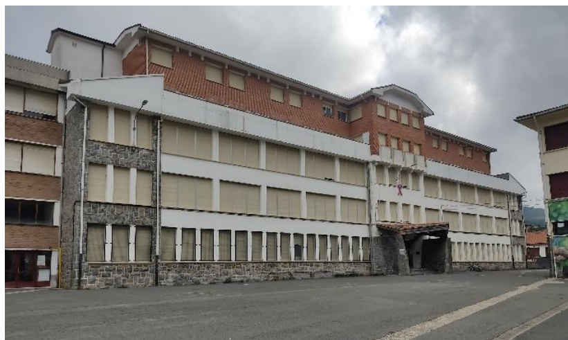
Figure 11. DS8 - school building
