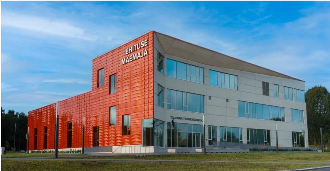
Figure 4. Demo Site 3 building outdoor view
