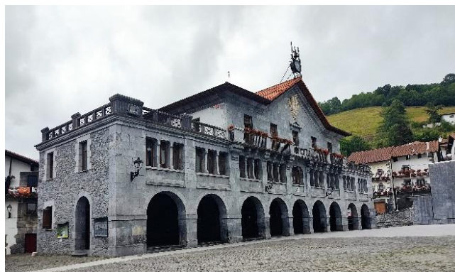
Figure 10. Exterior view of the building DS7
