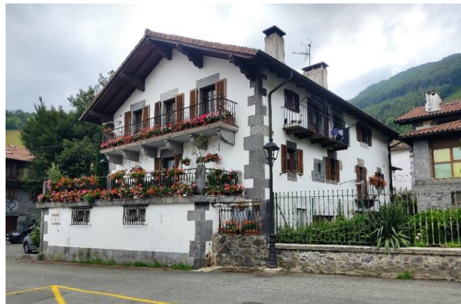
Figure 8. Exterior view of the building DS5
