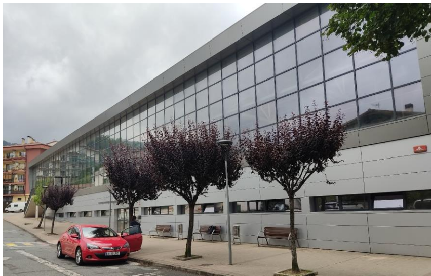
Figure 12. Exterior view of the building DS9
