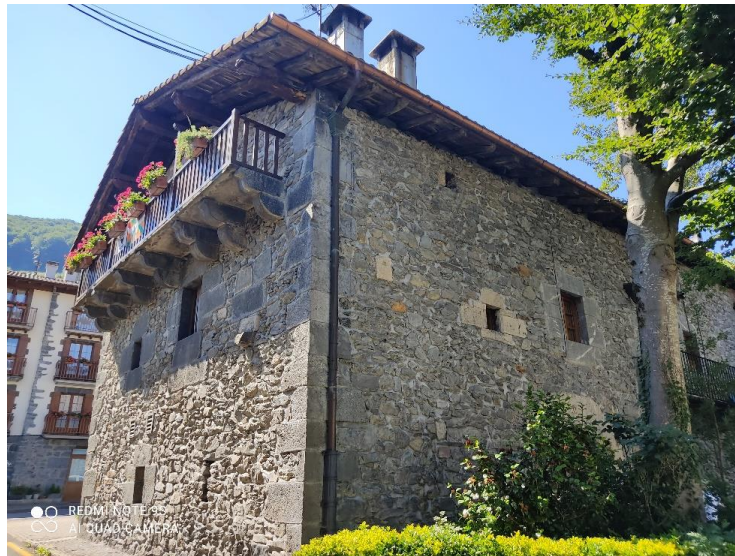
Figure 9. Exterior view of the building DS6
