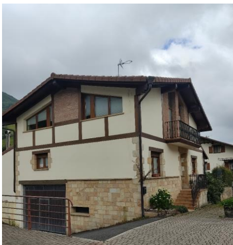
Figure 7. Exterior view of the building DS4
